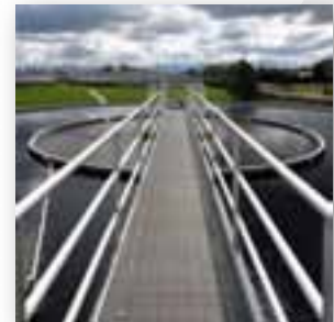
Potable Water Treatment
