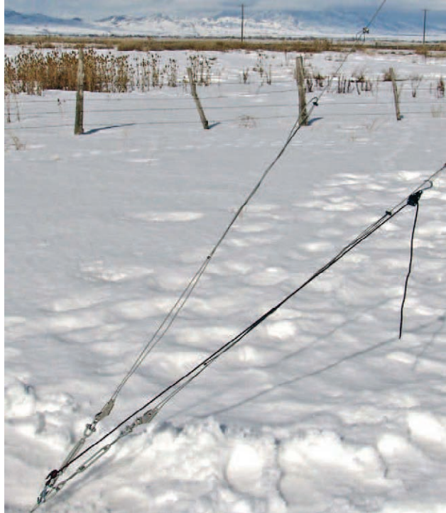
FIGURE 3-27. Rope ratchet assists assembly
